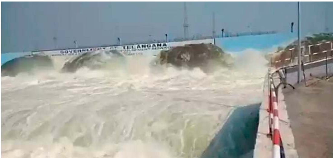
The water that is lifted from Gayatri pump house through four Bahubali motor pump sets here in Ramadugu mandal of Karimnagar district.
