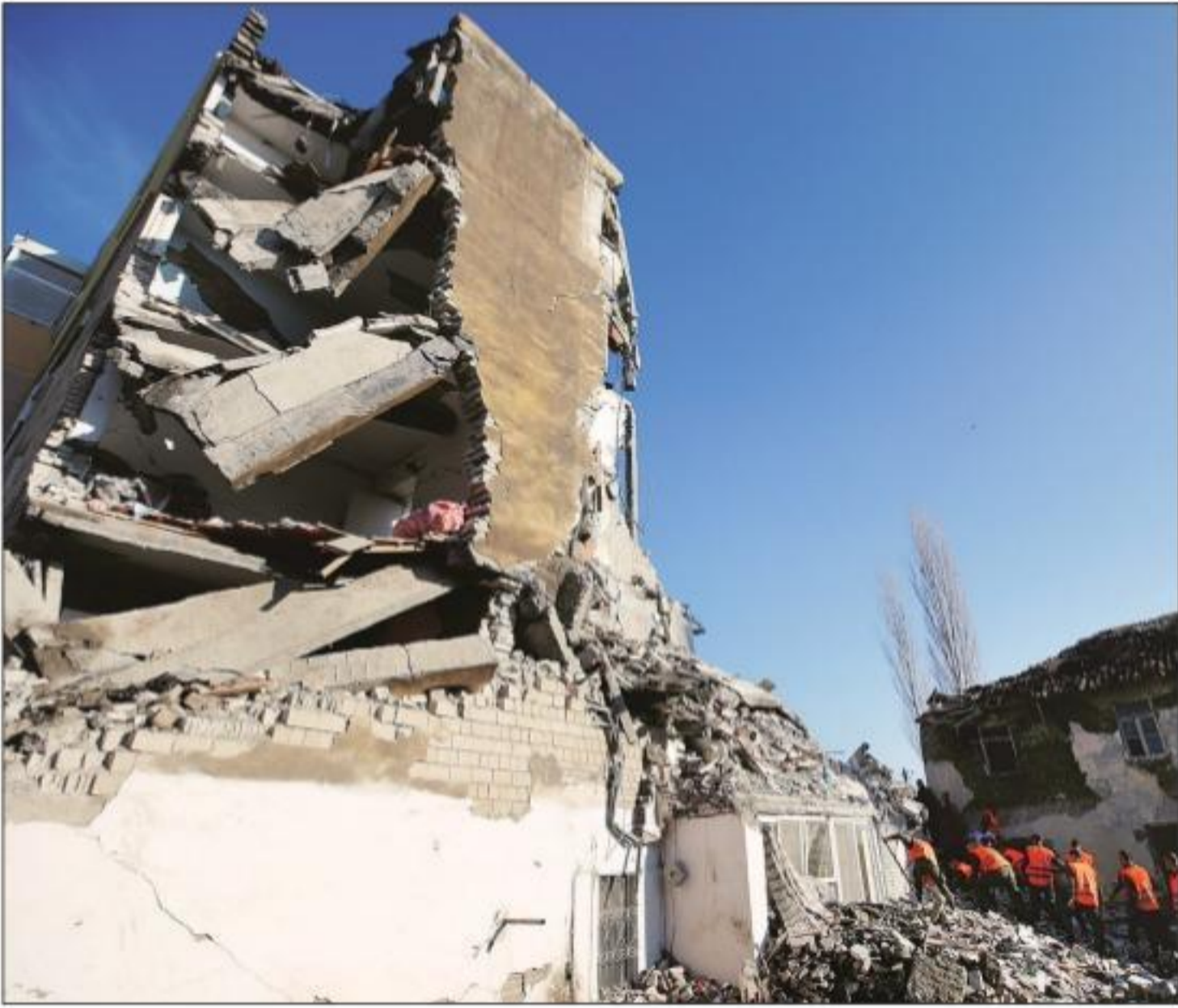
Emergency personnel work near a damaged building in Thumane, Albania, on Tuesday. Reuters
