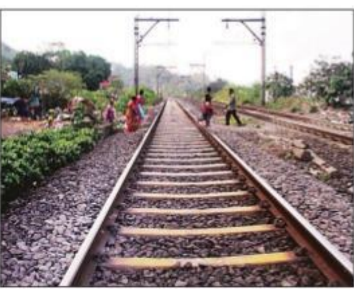
Sleepers painted yellow are part of innovation to prevent deaths on railway tracks. Deepak Joshi
