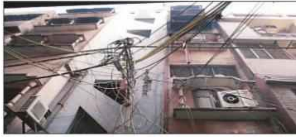
Three minors told police they had been employed on the second and third floors at manufacturing units in the building for the last six-eight months. Praveen Khanna
