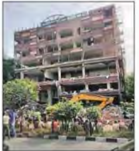
Hotel partly demolished while HC was hearing plea
