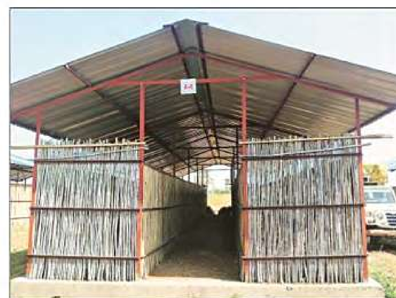
A typical 'Kanda Chawl' on-farm storage structure for onions. Express
