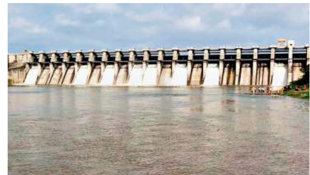
Urgent overhaul: An irrigation official said almost 70% of the Jayakwadi dam network needs major restoration. • FILE PHOTO
