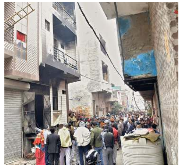
People gather outside the building in Kirari where a fire broke out in the early hours of Monday. •SHIV KUMAR PUSHPAKAR
