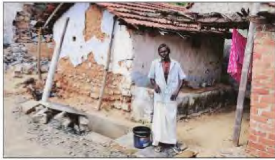
Subramanian outside his house near the spot where a wall collapse killed 17 Dalits in Mettupalayam. Arun Janardhanan
