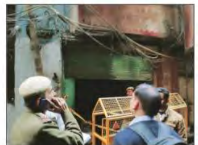
The shuttered entrance to the five-storey building. Express
