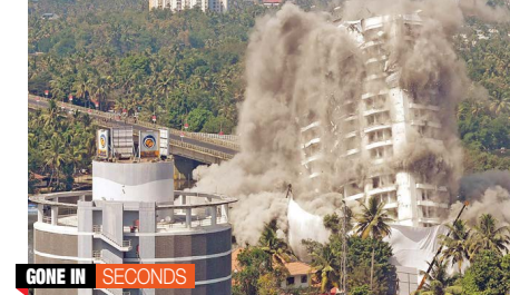
GONE IN SECONDS A view of Holy Faith H20, a water-front complex, being demolished using controlled implosion at Maradu in Kochi, on Saturday. REPORT ON P7
