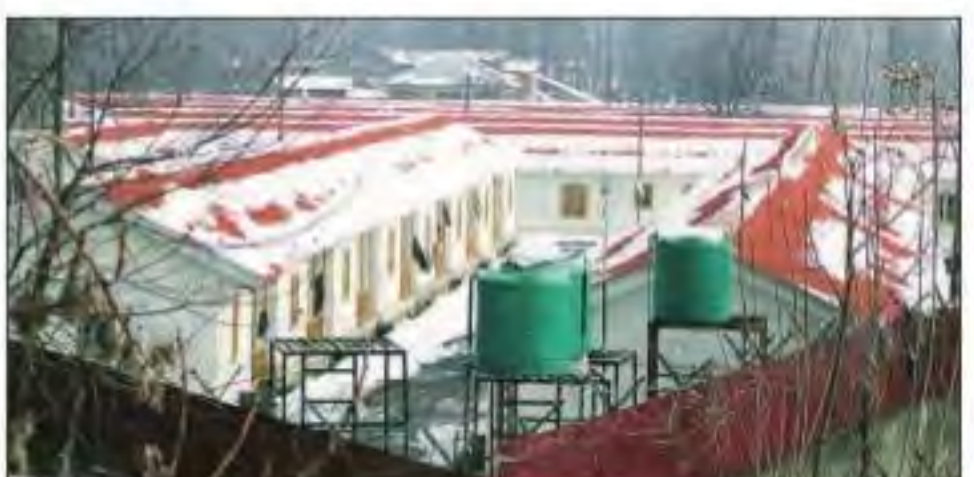
The gated colony at Haal in south Kashmir's Shopian houses around 70 families. Shuaib Masoodi
