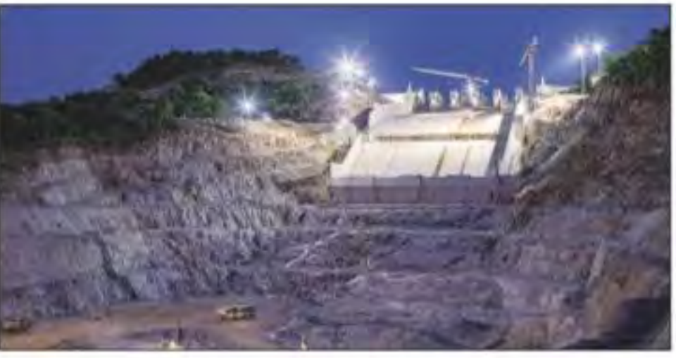
The Grand Ethiopian Renaissance Dam, under construction on the Blue Nile in Ethiopia. NYT
