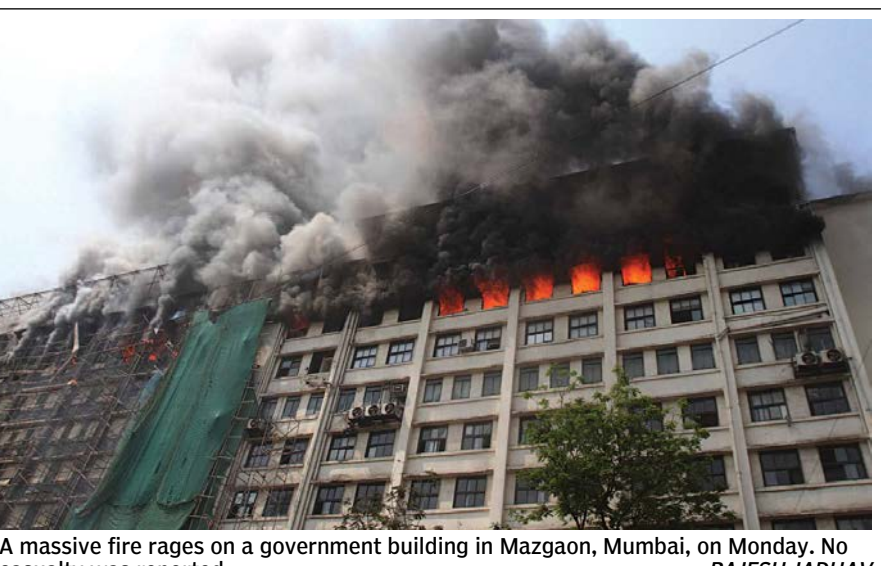
A massive fire rages on a government building in Mazgaon, Mumbai, on Monday. No casualty was reported. — RAJESH JADHAV
