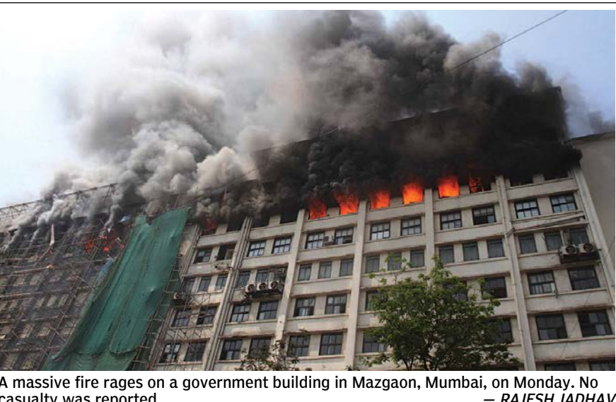
A massive fire rages on a government building in Mazgaon, Mumbai, on Monday. No casualty was reported. — RAJESH JADHAV
