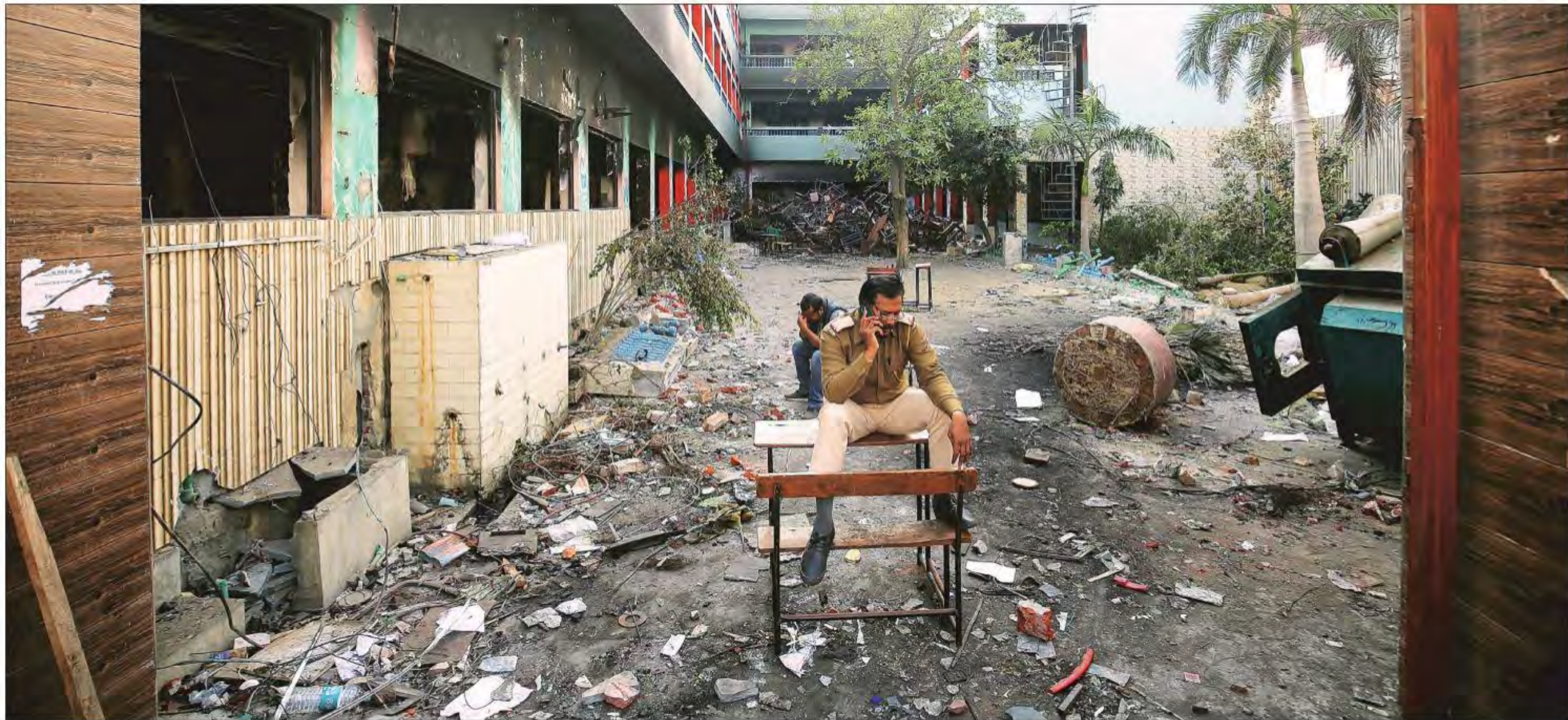
A school in Mustafabad that was targeted during the violence in Northeast Delhi. Several public properties suffered damage in the violence. Praveen Khanna
