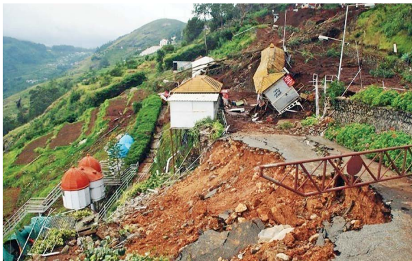
Destruction caused by Ooty landslide at Valley View point along Ooty NH in 2009. —DC
