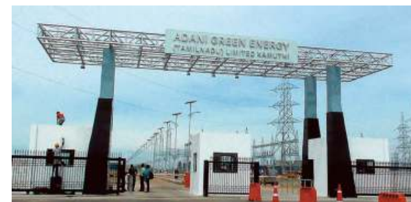
The solar portfolio of Adani Green Energy Limited is spread across 11 States in the country. ■ SPECIAL ARRANGEMENT
