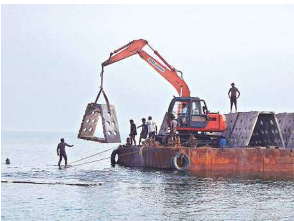
▼ (Below) Artificial reef modules being deployed; a view of deployed artificial reef modules; a researcher fixing PVC frames tied with seagrass shoots on the sea floor; researchers involved in the transplantation of seagrass shoots with jute rope
