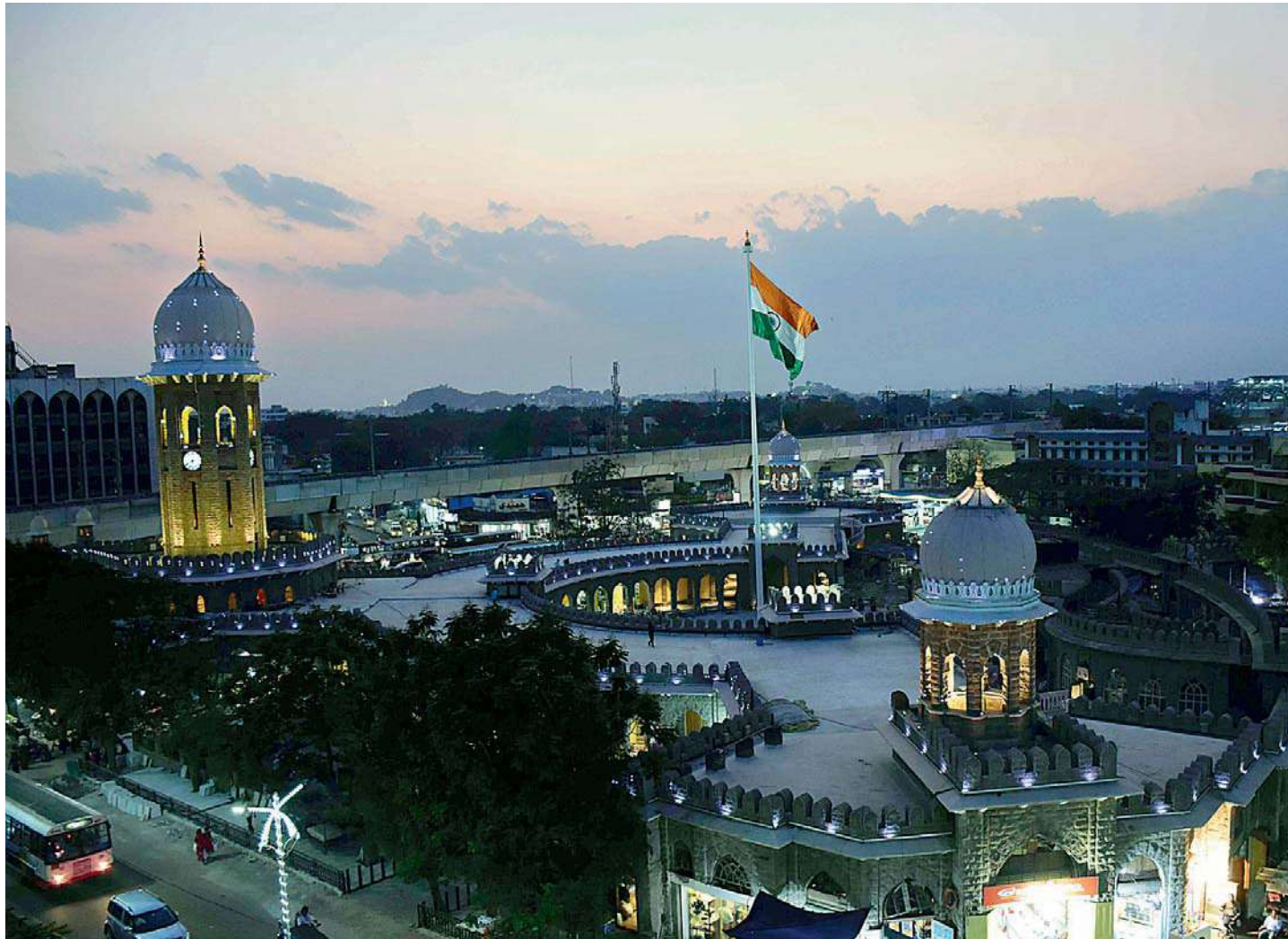
The Moazzam Jahi Market which is being renovated, looks resplendent in the evening.
