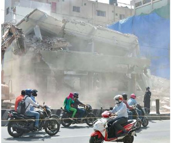
A view of the building demolished at Karkhana on Sunday night.
