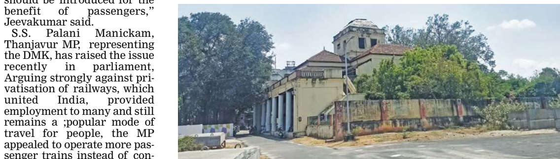
The first bungalow annexed by southern railway at Thanjavur. Now it is functioning as a health centre.
