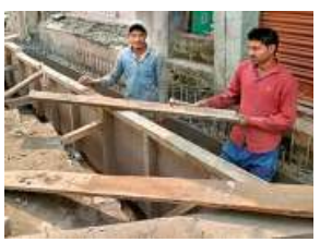
Workers engaged in a drainage project in Guwahati. • SPECIAL ARRANGEMENT
