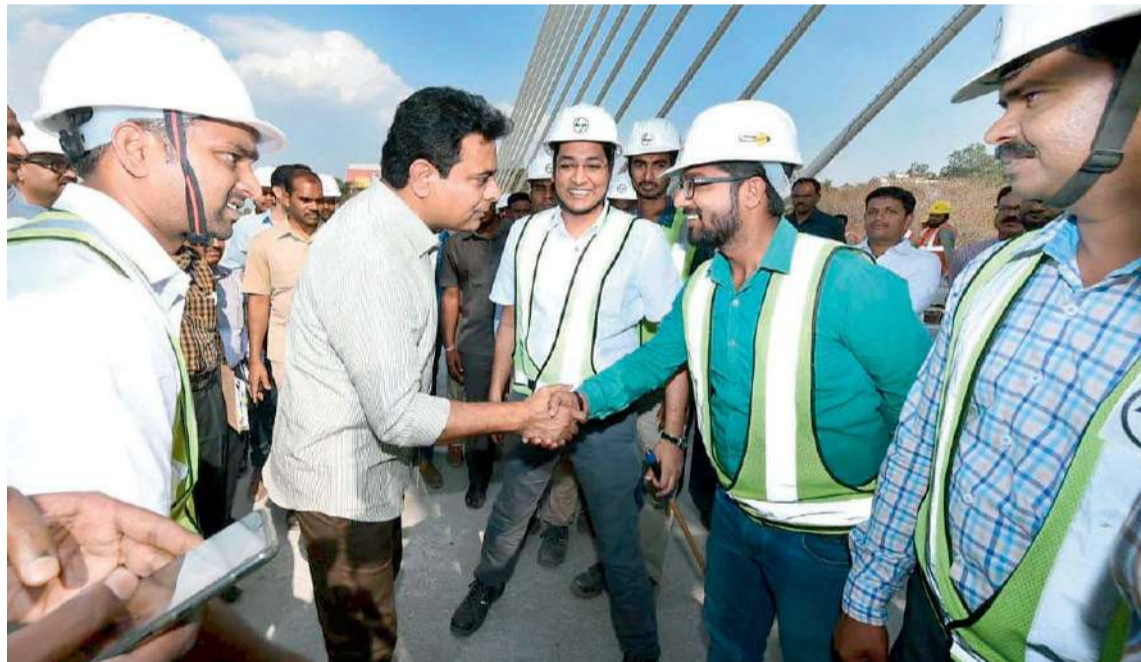
Municipal administration minister K.T. Rama Rao meets officials during his surprise visit to check the progress of the Durgam Cheruvu cable-stayed bridge work on Monday.
