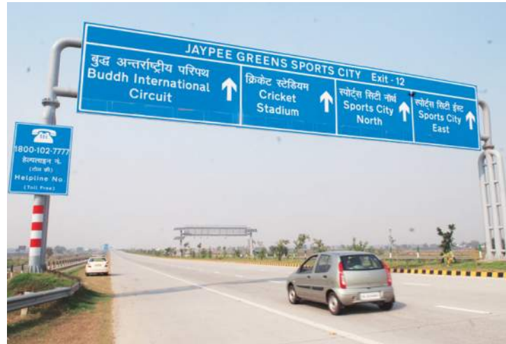
Jaypee Infratech has development rights over a land parcel of 6,175 acres along the Yamuna Expressway
